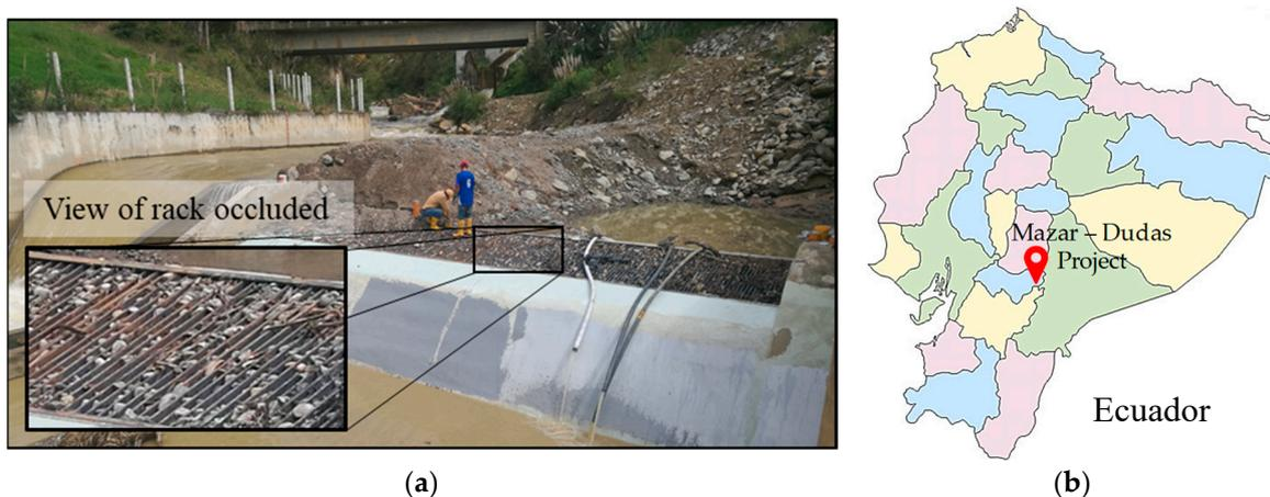
**Figure 2.** Mazar–Dudas Hydroelectric Project: (a) San Antonio bottom rack intake embedded in a weir—cleaning tasks and repairing process after a flood in the Mazar River, Ecuador (Image courtesy of Corporación Hidroeléctrica del Ecuador-CELEC EP Hidroazogues) [3]; (b) project location in Ecuador (without scale).
