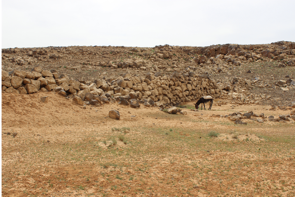
Figure 3. The Jawa dam, with the interior of the dam facing the viewer. Note the donkey for scale. © Bernd Müller-Neuhof (DAI-Orientabteilung), used by permission.
