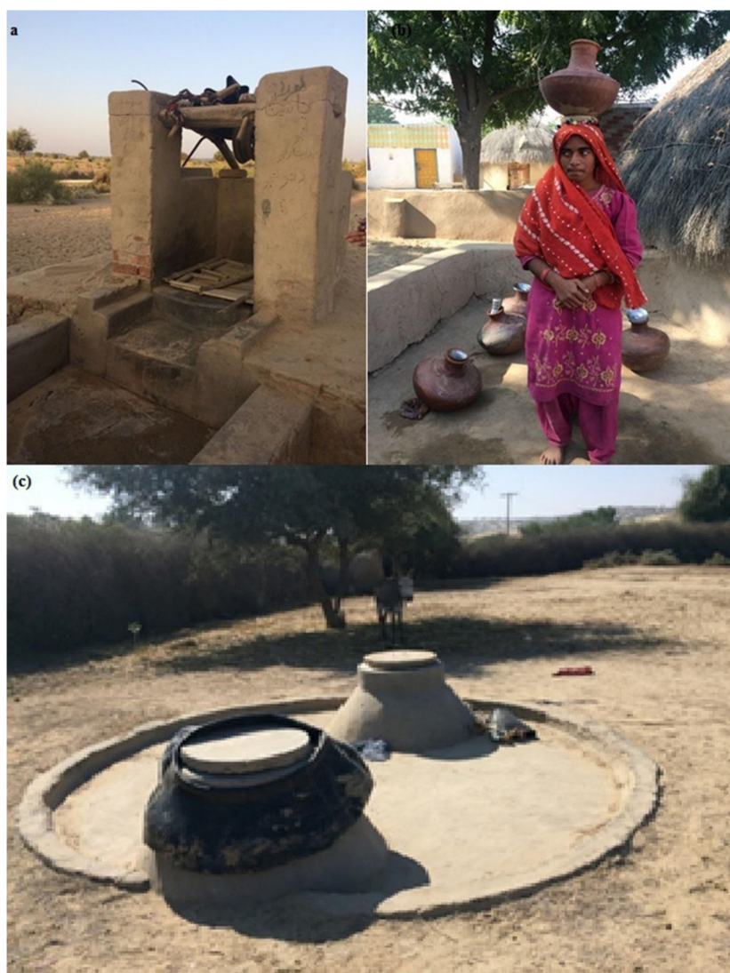
Figure 3. (a) Water wells, (b) Women carrying the mud container to fetch water, (c) Rain water storage containers “TARAIIS”.
