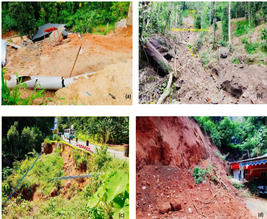
Figure 2. Damages that happened due to landslides in the Idukki district in 2018. (a) Debris slide at Anachal. (b) Debris flow at Kallimai. (c) Subsidence at Kallarkutty approach road. (d) Earth slide at Cheruthoni [22].
