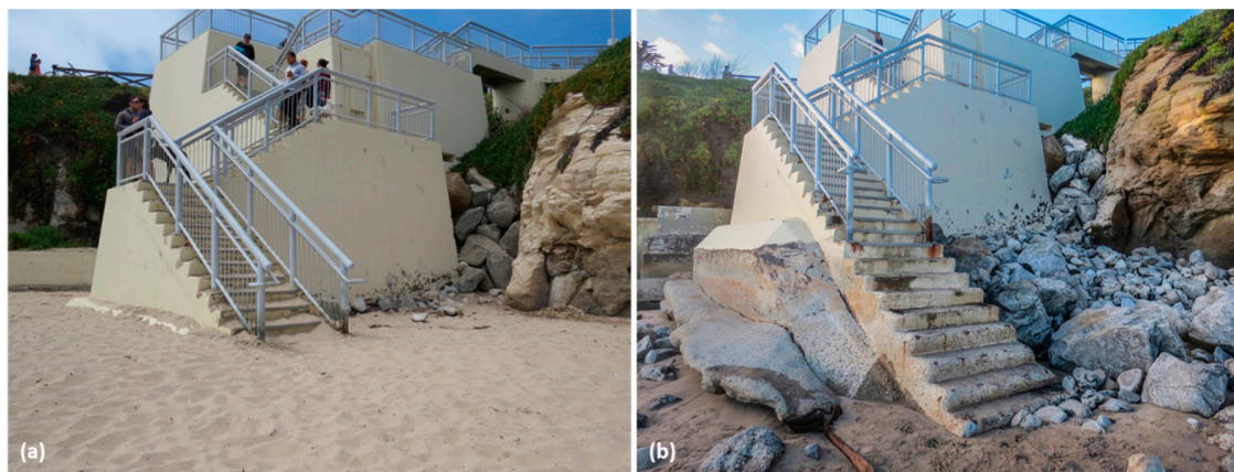
Figure 8. (a) Summer and (b) winter beach sand levels along West Cliff Drive (photos by Gary Griggs).
