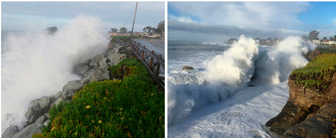
Figure 7. Storm waves at high tide overtopping West Cliff Drive bluff (photos by Gary Griggs).
