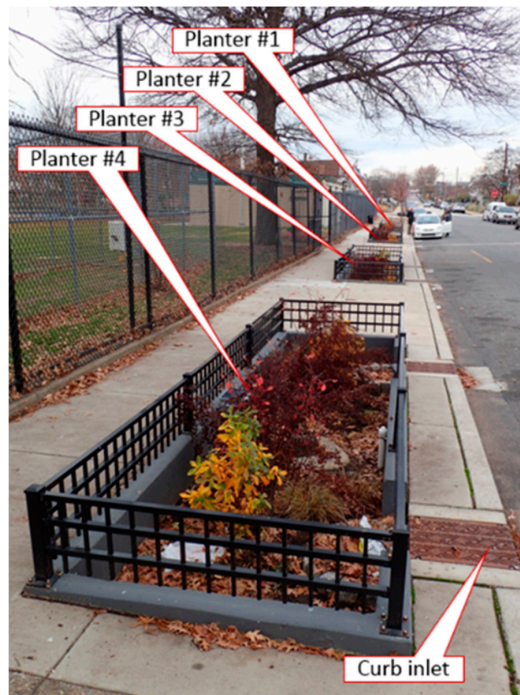
Figure 1. Green infrastructure sidewalk planters under investigation (reprinted from Tu and Traver [22] with permission from ASCE).
