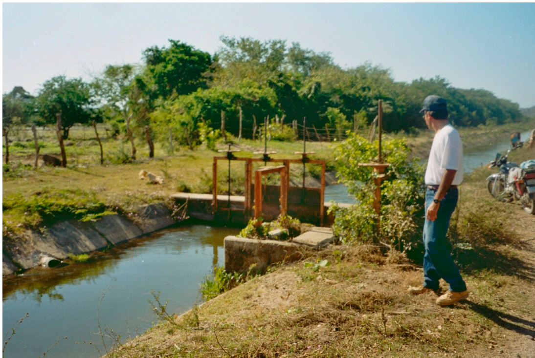
Figure 4. The canalero near a cross-regulator and intake structure.
