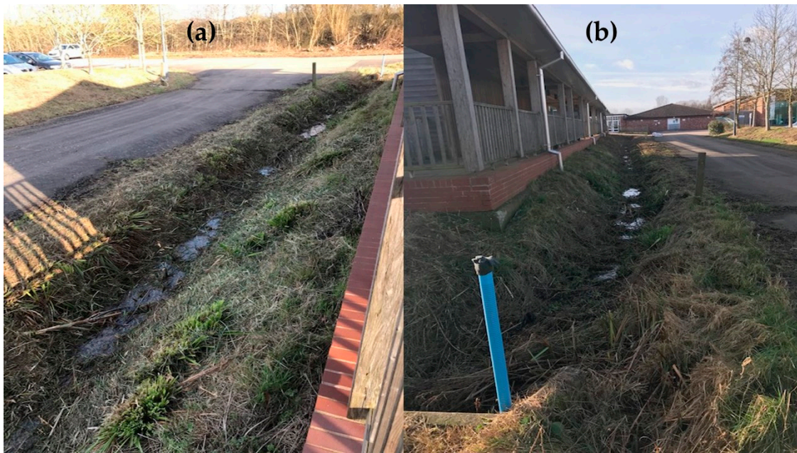
Figure 5. Detail of the swale after complete removal of vegetation (February 2020): (a) South-west sight of the swale; (b) North-east view of the swale from the discharge point and the monitoring device.
