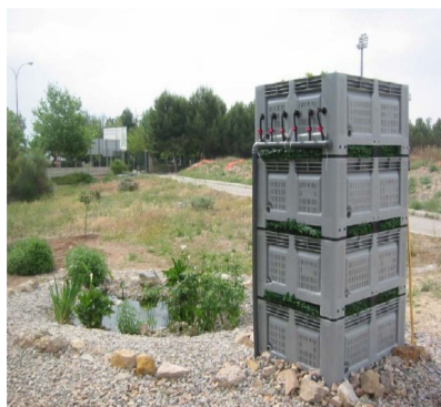
Figure 4. Picture of the pilot plant with vertical arrangement.
