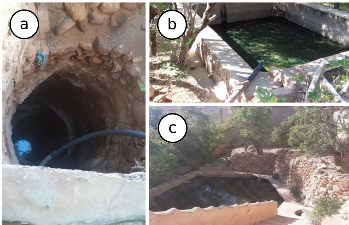
Figure A3. Nodes of the irrigation system. (a) A well with mechanical pump. (b) A modern and recent reservoir. (c) A traditional reservoir.
