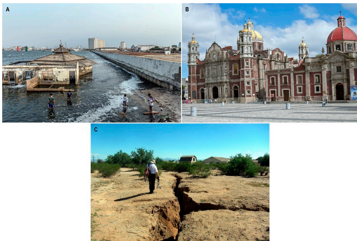
Figure 2. Adverse effects of over-exploitation of groundwater: (A) the increase in the risk of flooding in Jakarta; the combined effects of both land subsidence and the increase in the average ocean level caused the need to build a sea wall to protect the city from floods, especially during stormy periods (photo credit by Graham Crouch [55]); (B) the twist and deformation of surface infrastructure in Mexico City; some buildings have been deemed unsafe and have been closed, and many others have needed repairs to keep them intact; land subsidence affected historic urban areas, including the Metropolitan Cathedral (photo credit by Czuber [56]); (C) an earth fissure in a farmland area of Chandler Heights, Phoenix, Arizona (courtesy of the Arizona Geological Survey, photo by Joseph Cook [57]).
