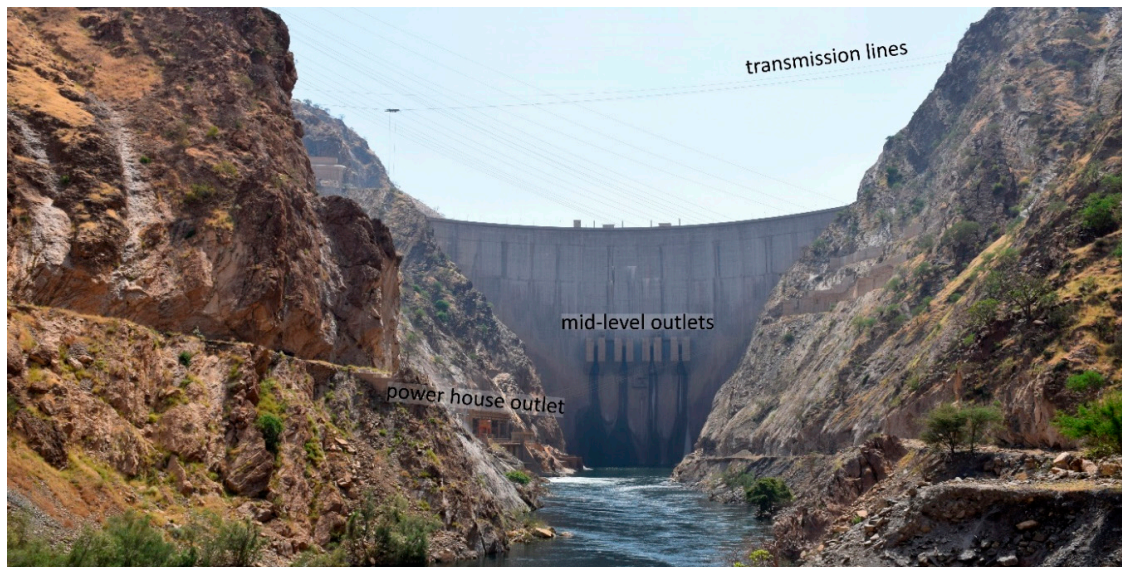
Figure 8. Downstream view on the 188 m high Tekeze arch dam with its four mid-level outlets and transmission lines crossing the narrow gorge (Photo: 15 October 2018).
