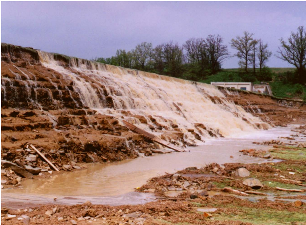
Figure 11. Overtopping of the Pocheň dam in 1996.
