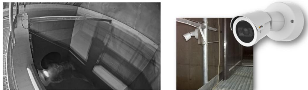
**Figure 11.** IR camera with an image of the forebay tank emptied.
