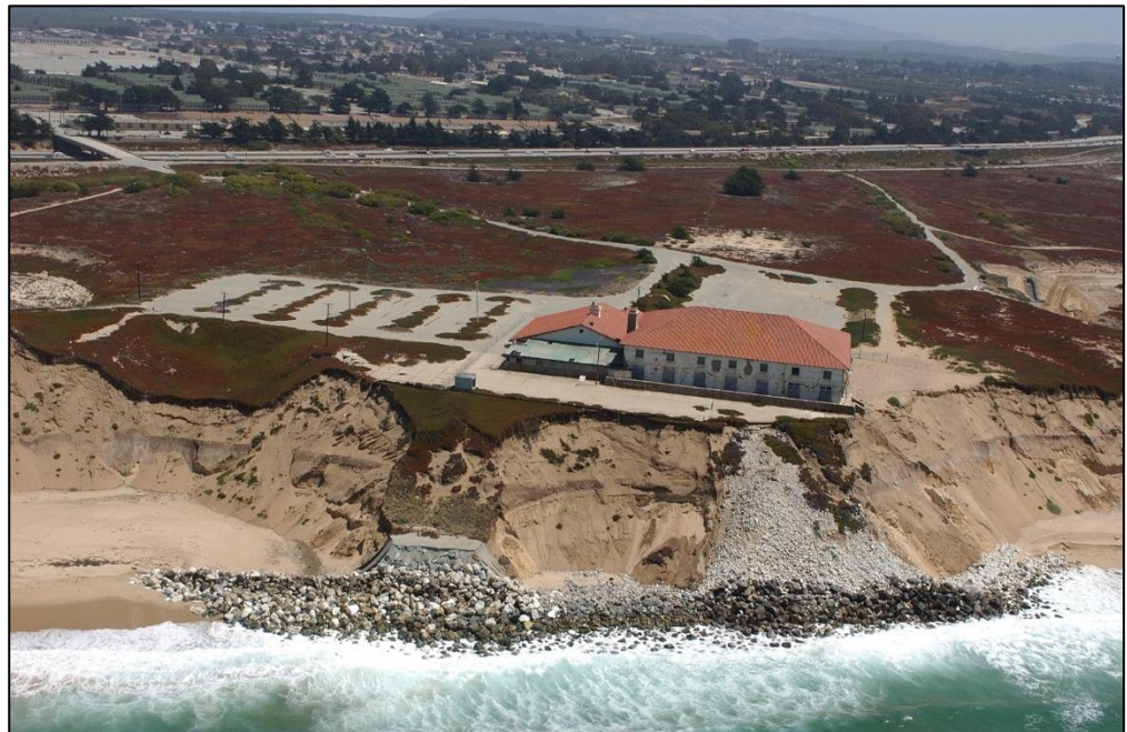
Figure 12. Passive erosion (loss of beach) in front of a rock revetment in central Monterey Bay, California, while a beach continues to exist on either side where there is no armor. Courtesy: California Coastal Records Project.
