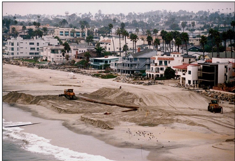
Figure 11. A number of beaches on the northern San Diego County coastline, California, have been nourished twice with a total of 2.7 million m 3 of sand at a total cost of USD 46 million. Beach surveys showed most of the sand had moved downcoast with littoral drift with a year or two (Courtesy: SANDAG Regional Beach Sand Project).
