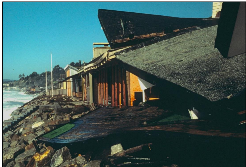
Figure 5. Storm waves arriving simultaneously with high tides broke through the front of these homes built along the northern Monterey Bay, California, shoreline (Photo: Gary Griggs).
