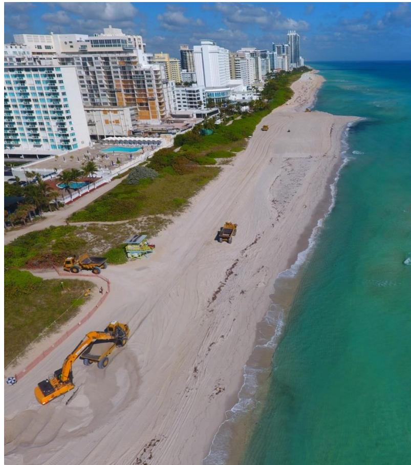
Figure 10. The U.S. Army Corps of Engineers dumps new sand from Central Florida (USA) along the Miami Beach shoreline. Source: U.S. Army Corps of Engineers.
