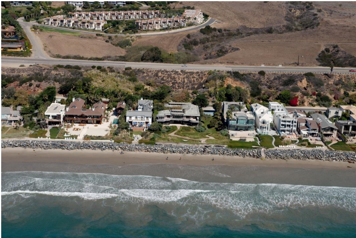
Figure 4. Rip-rap revetment armoring a section of the Malibu, California (USA) shoreline. Courtesy: California Coastal Records Project.
