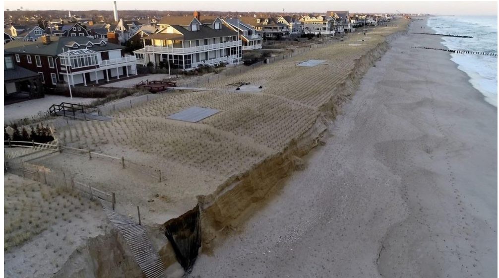
Figure 14. Storm waves along the U.S. Atlantic coast have removed a major portion of a newly built and vegetated dune at Bay Head, New Jersey (Photo: Mike Davis and Thomas P. Costello).
