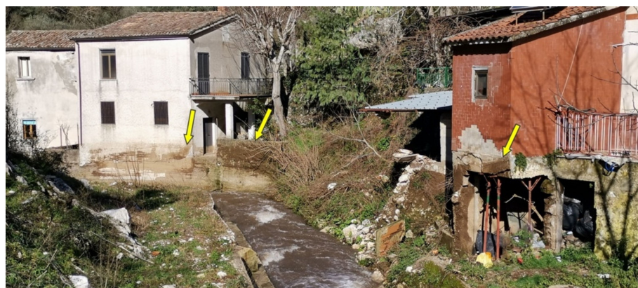
Figure 12. View of Caudino Torrent downstream of the first covered segment (cf. Figure 6) and houses hit by the 2019 debris flow. The indicators of the flow thickness are shown by the arrows.
