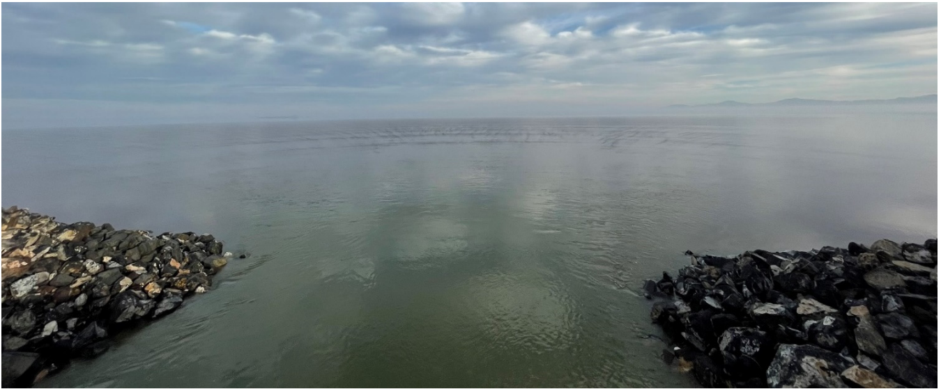
Figure 11. View from the WC breach at the Great Salt Lake Causeway looking north. Surface flows move from south to north (bottom to top of photo). Note the radial pattern at the surface, providing indication of the relatively lighter water from the south floating over the heavier northern water. Similar radial mixing patterns at the surface can also be observed in the CFD simulation (see Figure 12).
