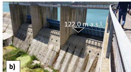
Figure 2. Upper panel: surface spillway, bottom outlet components and dissipating structures. Lower panel: surface spillway: (a) ungated ogee weir (free Creager type sill); (b) gated weir with three 13 m wide openings, equipped with automatic flap gates.
