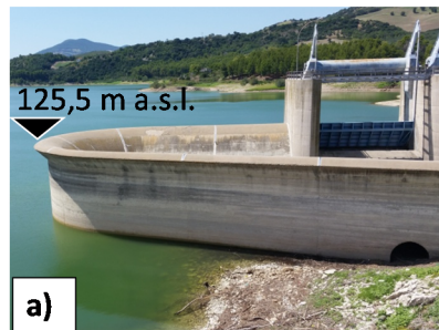
Figure 2. Upper panel: surface spillway, bottom outlet components and dissipating structures. Lower panel: surface spillway: (a) ungated ogee weir (free Creager type sill); (b) gated weir with three 13 m wide openings, equipped with automatic flap gates.
