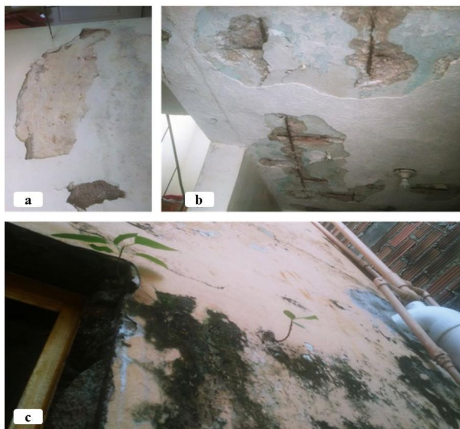
**Figure 4.** Single-family household obsolete plumbing installation affectations. (a) Interior dampness, (b) exposed structural reinforcement due to dampness, and (c) exterior dampness.
