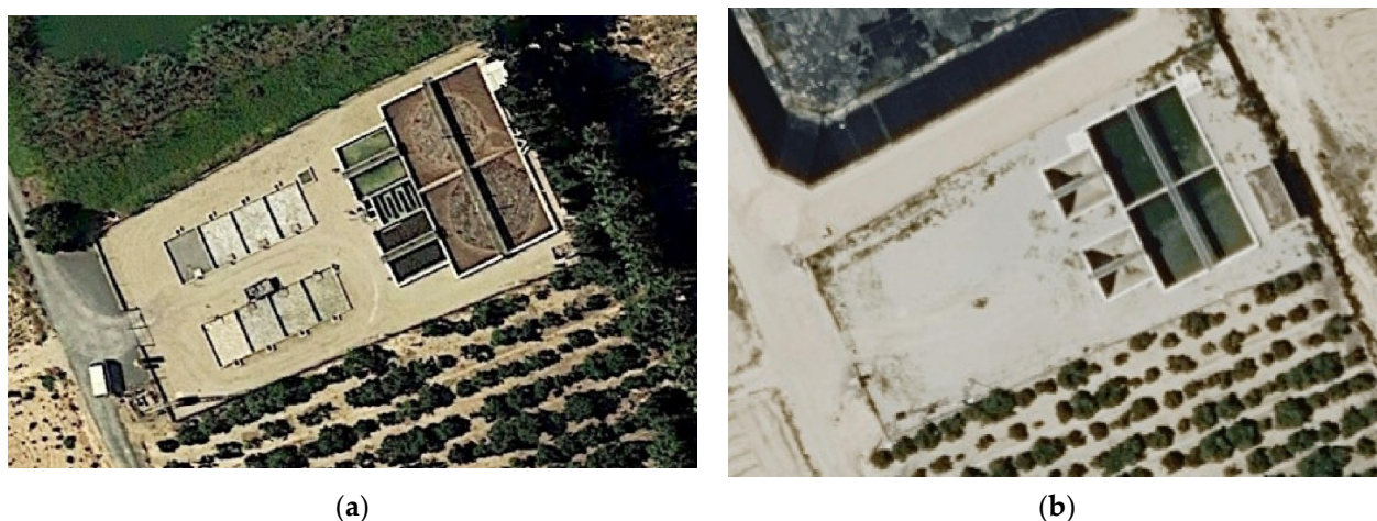
Figure 4. (a) Doña Pepa WWTP before its transformation; (b) Doña Pepa WWTP after transformation into a combined sewer system storm overflow tank. Source: (a) Google Earth (7 June 2018); (b) ICV (2021) (21 June 2021). Own elaboration.
