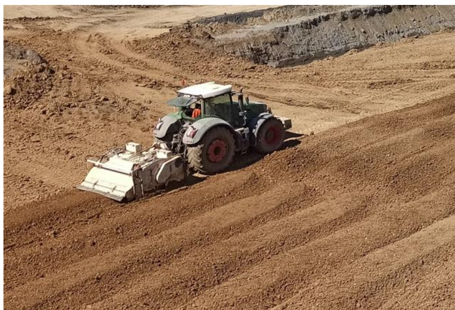
Figure 3. Mechanical drainage. A combination of stabiliser and tractor (photo: Michal Bernacki).
