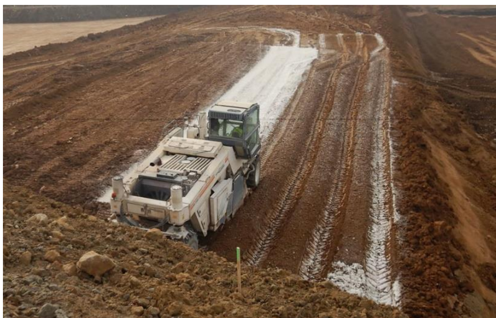
Figure 4. Lime stabilisation. MPH 600 recycler (photo: Michal Bernacki).
