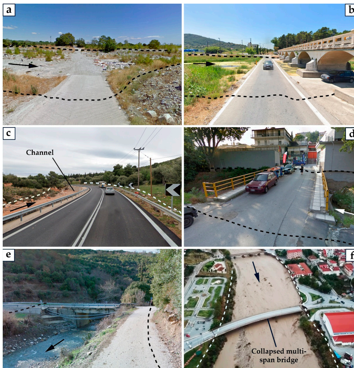
Figure 2. Typical examples of infrastructure in locations where people lost their lives, including (a) an unimproved ford crossing, (b) an improved but unvented ford crossing, (c) an asphalt road beside a river channel, (d) a low water bridge, (e) a single-span bridge and (f) a collapsed multi-span bridge. The dashed lines and the arrows denote the approximate maximum extent of the inundated area during the event under study and the direction of flow, respectively. All the locations shown were included in the present study.
