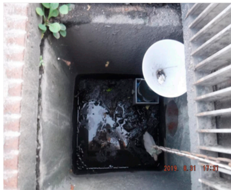
Figure 2. Inside the street stormwater inlet.
