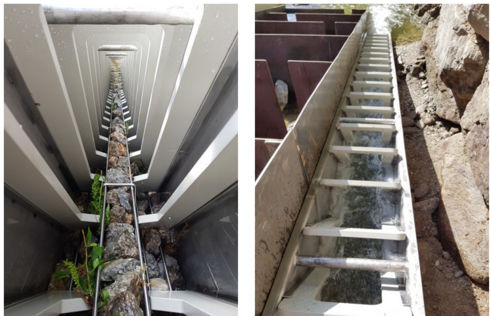
Figure 4. (Left): baffle geometry and substrate gabion. (Right): modified Denil fishway (MDF) in operation.
