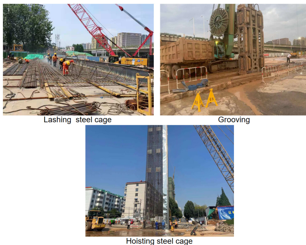
Figure 5. Construction picture of underground diaphragm wall.
