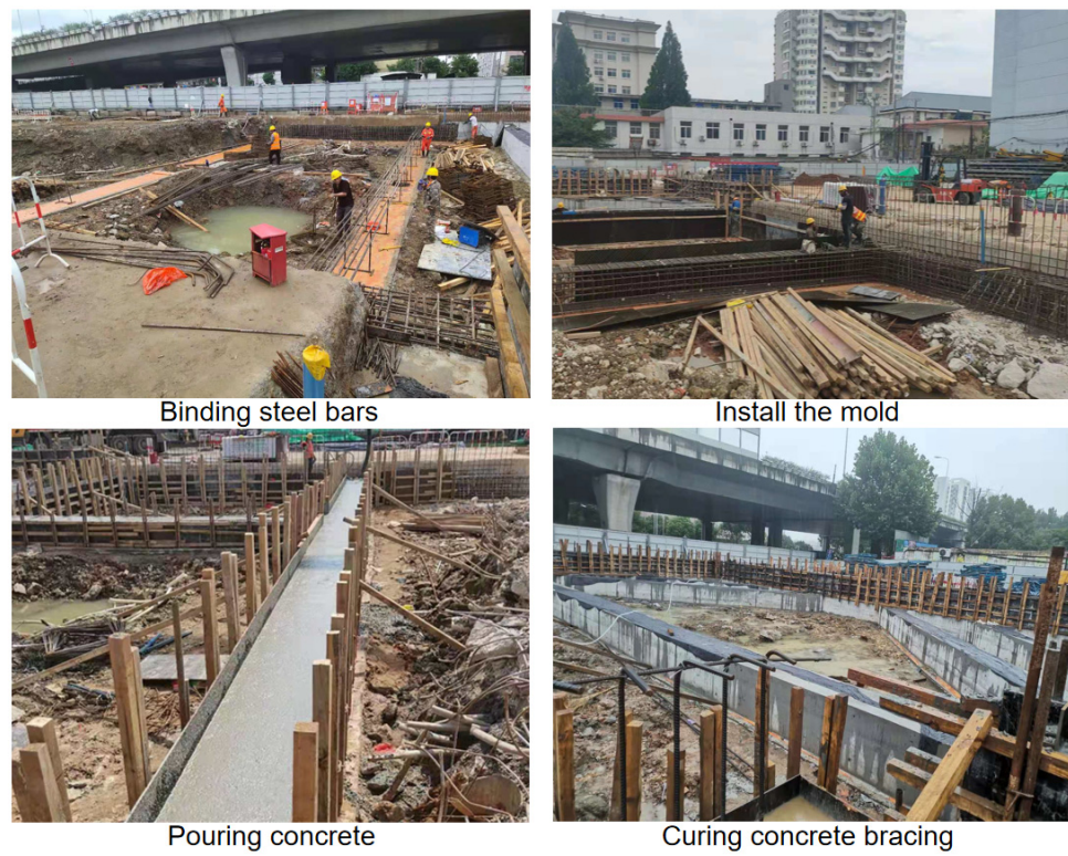
Figure 13. Construction process of the first reinforced concrete internal bracing.
