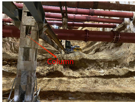
Figure 17. The construction picture of the column.
