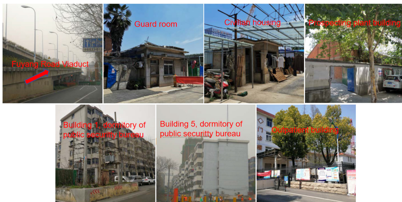
Figure 2. Fuyang Road viaduct and buildings around the foundation pit.
