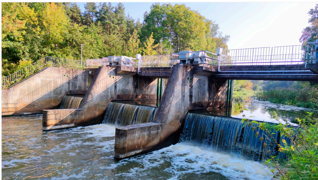
Figure 8. Concrete weir on Świder river (downstream view) (Authors' property).
