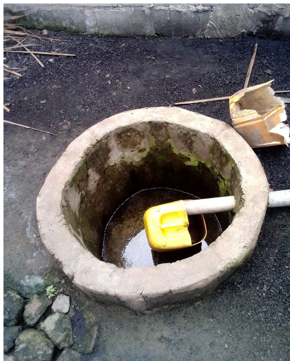
Figure 7. Wastewater reservoir in the center of Adétikopé (field photo, CEESPOD, December 2022).
