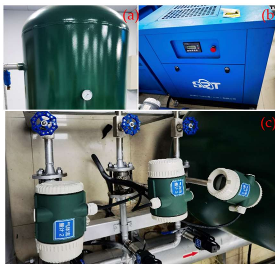
Figure 4. Physical picture of the gas supply module unit: (a) gas storage tank; (b) air compressor; (c) vortex gas flow meter.
