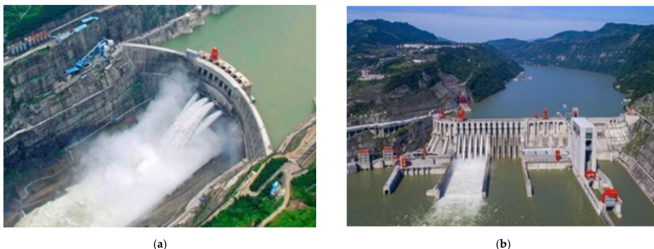
Figure 1. Typical high concrete dams: (a) Xiluodu arch dam and (b) Xiangjiaba gravity dam.
