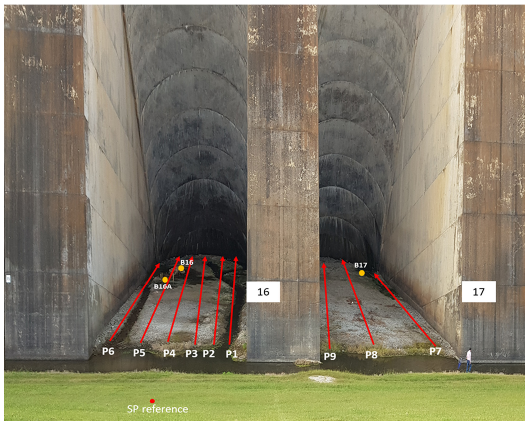
Figure 6. Location of the acquired ERT, SP, and seismic P-wave refraction geophysical profiles and borehole inside Arch-16 and Arch-17 at Pensacola Dam. The orange dot represents the boreholes. Not drawn to scale.
