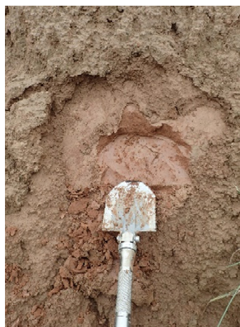
Figure 5. Silty clay in the landslide site.
