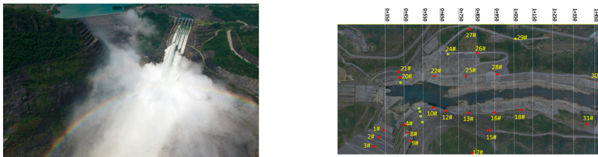
Figure 10. FDA scene and atomization rain intensity monitoring points of Shuibuya Hydropower Station.
