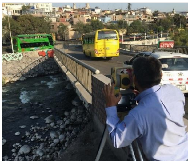
Figure 1. Surveying of the bridge.
