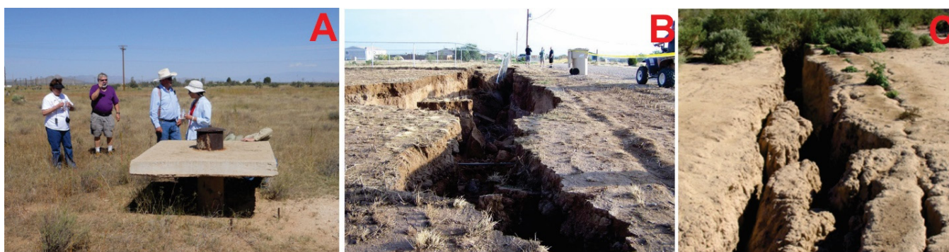
Figure 5. The effects of land subsidence in the area of Arizona. (A) Max vertical deformation reached 75 cm between 1940–1950 [79]. (B) Surface ruptures were reopened after a major rain in August 2005 [77]. (C) Surface ruptures [80].
