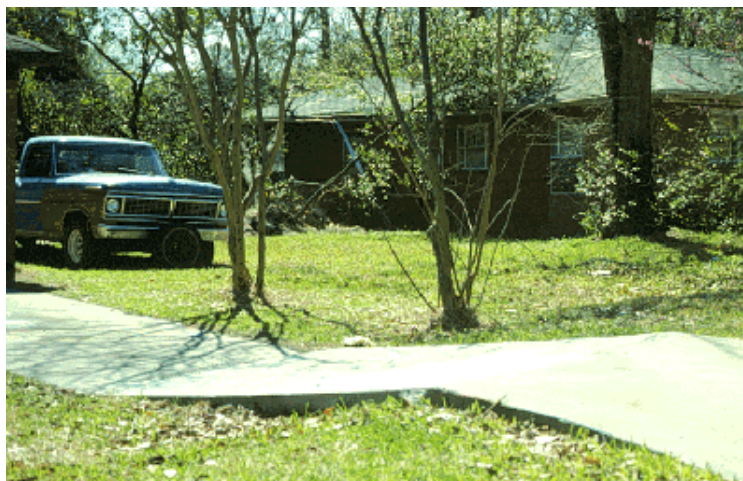
Figure 4. Land subsidence in the area of Pasadena [69].
