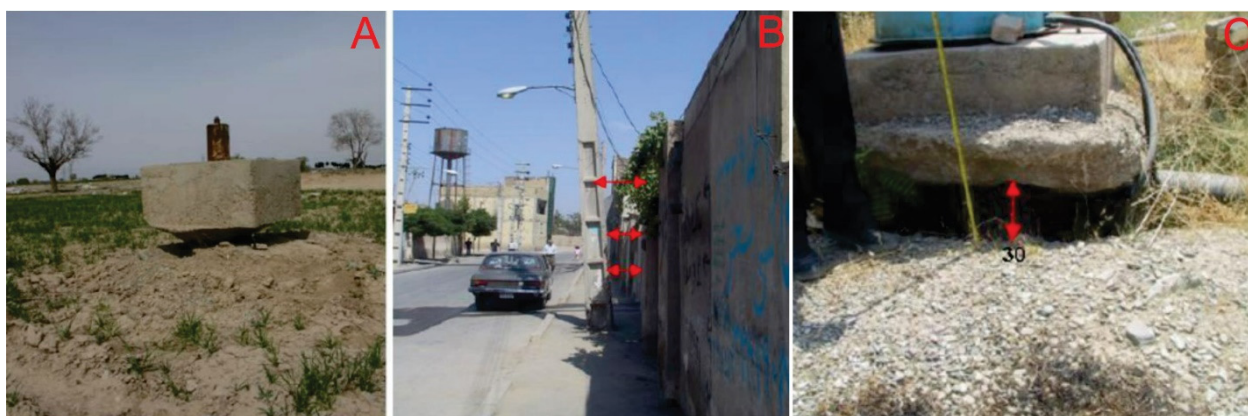
Figure 11. Damages due to the overexploitation of the aquifer in Tehran: (A) uplifting of boreholes (Sabashahr). (B) damage to the electricity network red arrows showing the deviation from the vertical (Sabashahr). (C) Damaged boreholes suggesting a drop of 30 cm (Eslamshahr and Ahmadabad) [193].
