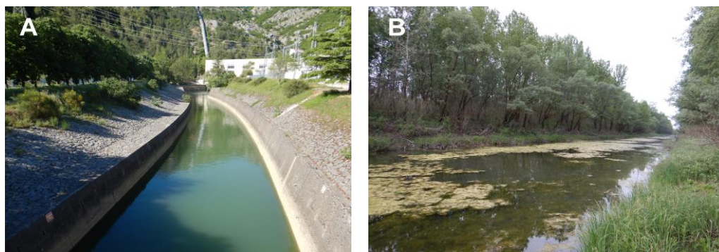
Figure 7. Artificial water bodies: outflow from the HPP (A) and flood-protection canal with good morphological conditions (B).
