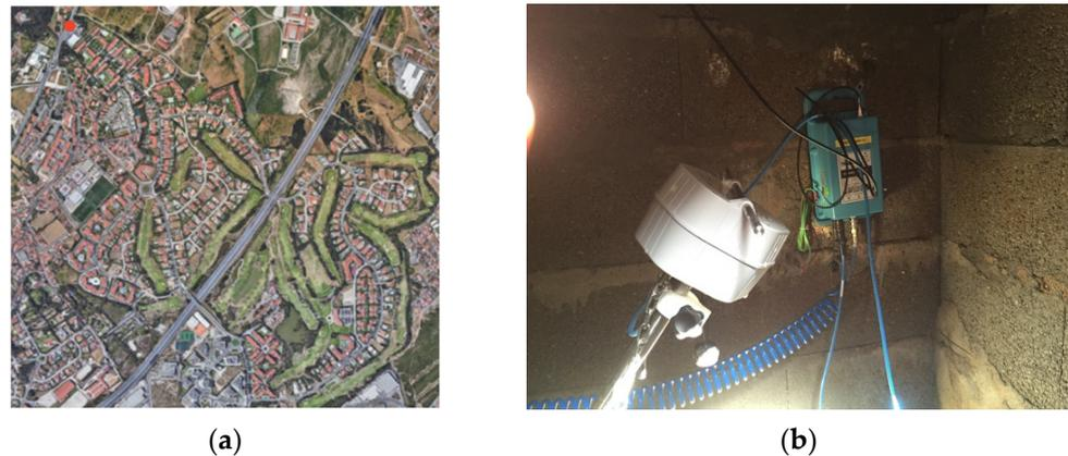
**Figure 6.** Aerial view of the Beloura DMA (a); flowmeter and data-logger (b).
