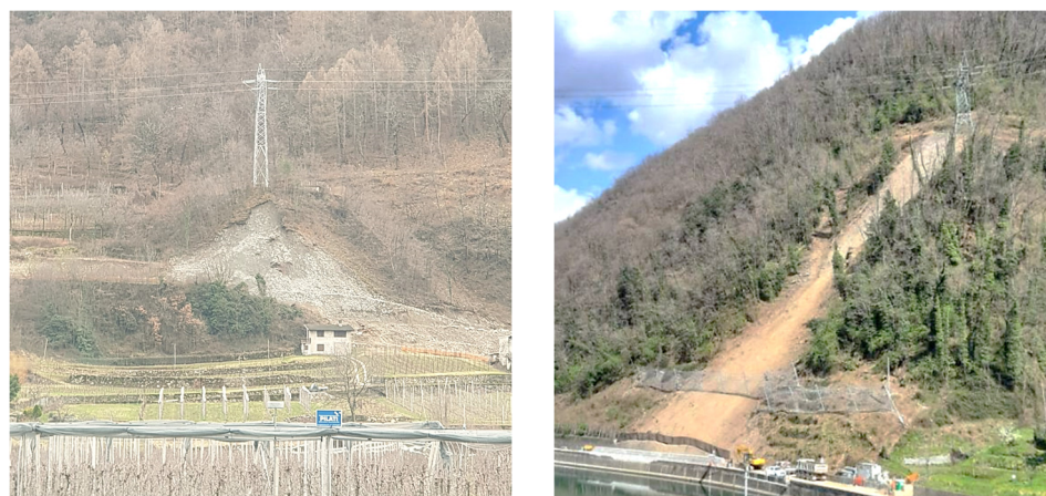
Figure 1. Powerlines affected by shallow landslides in their proximities: slope failure can trigger pylon collapse, causing blackouts.
