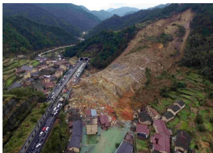
Figure 4. Top view of landslide damage.
