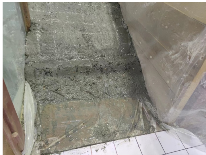
Figure 12. Water seeped out of the initial dam.
