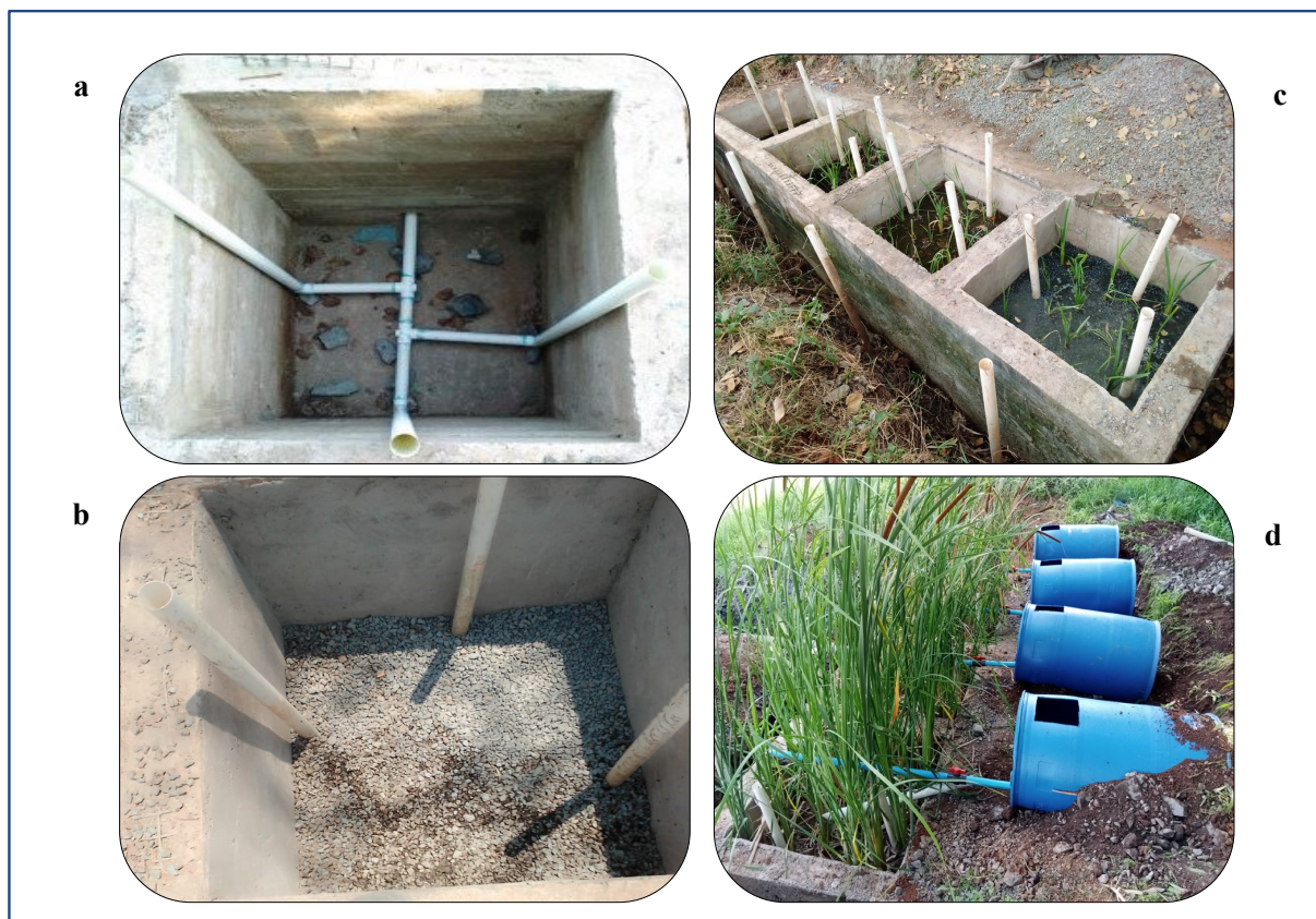
Figure 2. Layout of a VF CW. (a) Section of one unit showing the aeration pipe layout, (b) a unit being filled with rock pebbles, (c) four VF CWs, three planted with T. latifolia and one unplanted, and (d) a VF CW connected to reservoirs of raw sewage.
