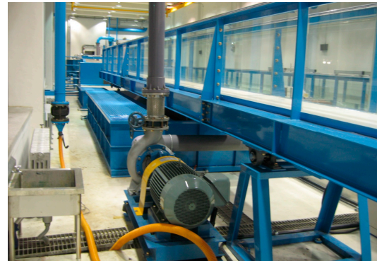
(b) Water supply pump
