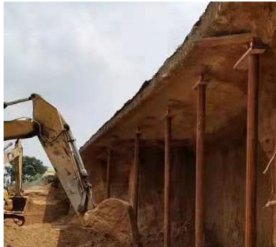
Figure 11. Crest hardening ensures “overtopping without breaking”.
