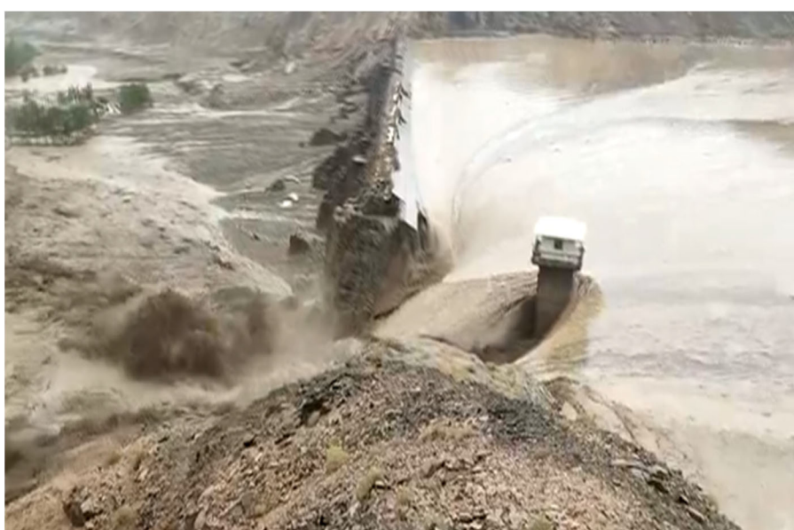
Figure 8. Overtopping and break of Sheyuegou Reservoir.
