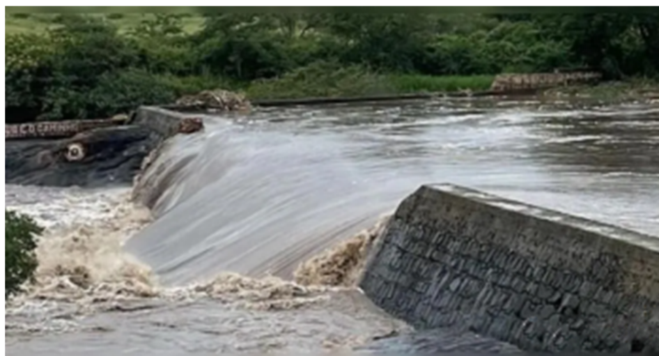
Figure 7. Breaking Jussiapé Dam.
