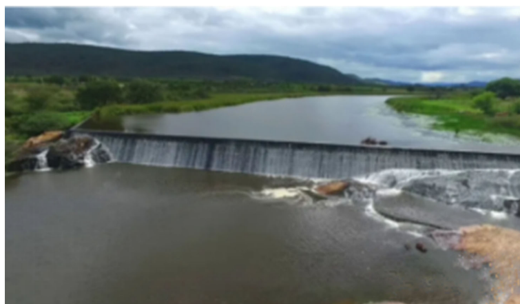
Figure 6. Jussiape Dam before break.
