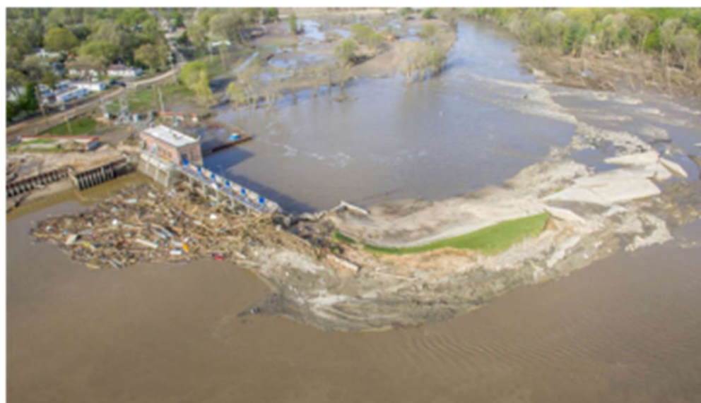
Figure 2. Aerial image of the Sanford Gate Dam.
