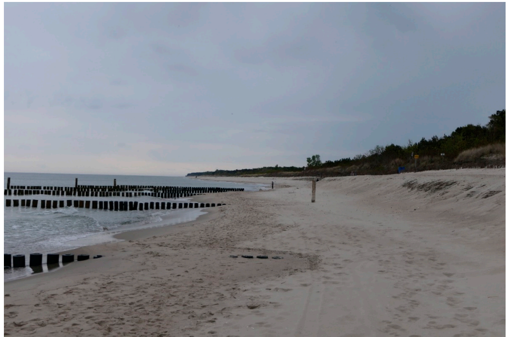
Figure 20. View of the endpoint of the newly constructed groyne group on the Hel Peninsula. In the distance, erosion of the coast and dune can be seen, located at km H 10.9. (Photograph taken on 21 May 2021, credited to P. Szmytkiewicz).
