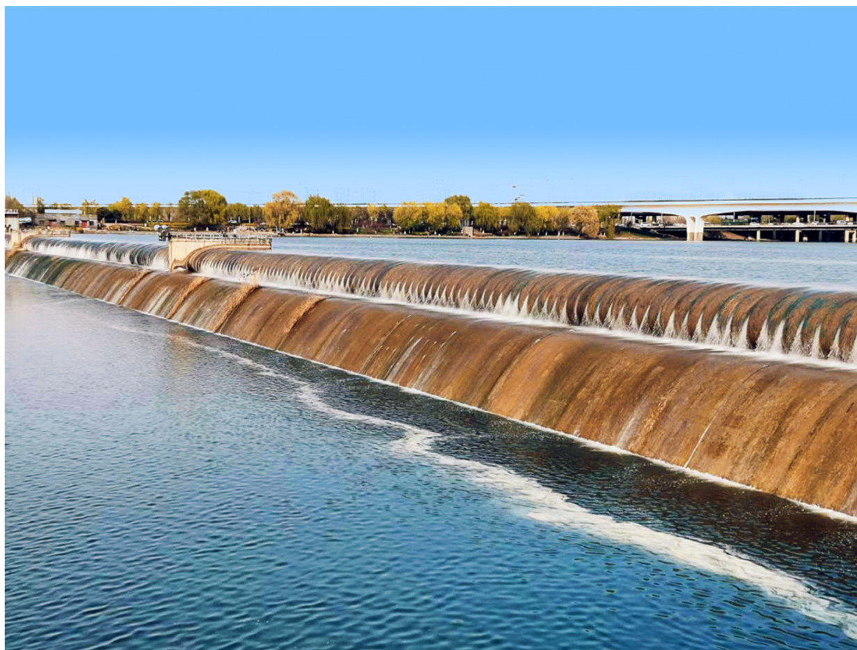
Figure 3. The image of rubber dam project.
