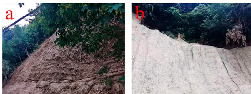
Figure 1. Schematic diagram of lead wire mesh and plant blanket. (a) Lead wire mesh, (b) plant blanket.
