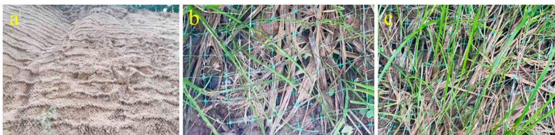
Figure 7. Composition of ecological restoration measures. (a) Hanging nets, (b) planting blankets, (c) vegetation recovery.
