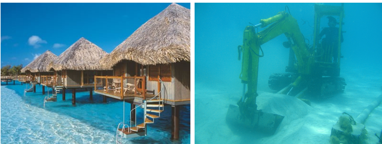
Figure 6. View of “motus” and the construction of the distribution network.
