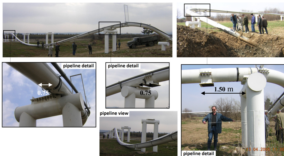
Figure 1. Pipeline accident (adapted from [23]).
