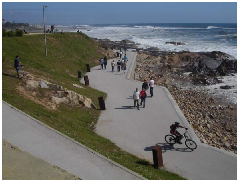
Figure 6. Detail of a submergible pathway that uses strong and resistant materials. More specifically Passeio Atlântico at Porto, Portugal. Image credits: Maria Matos Silva, 2007.
