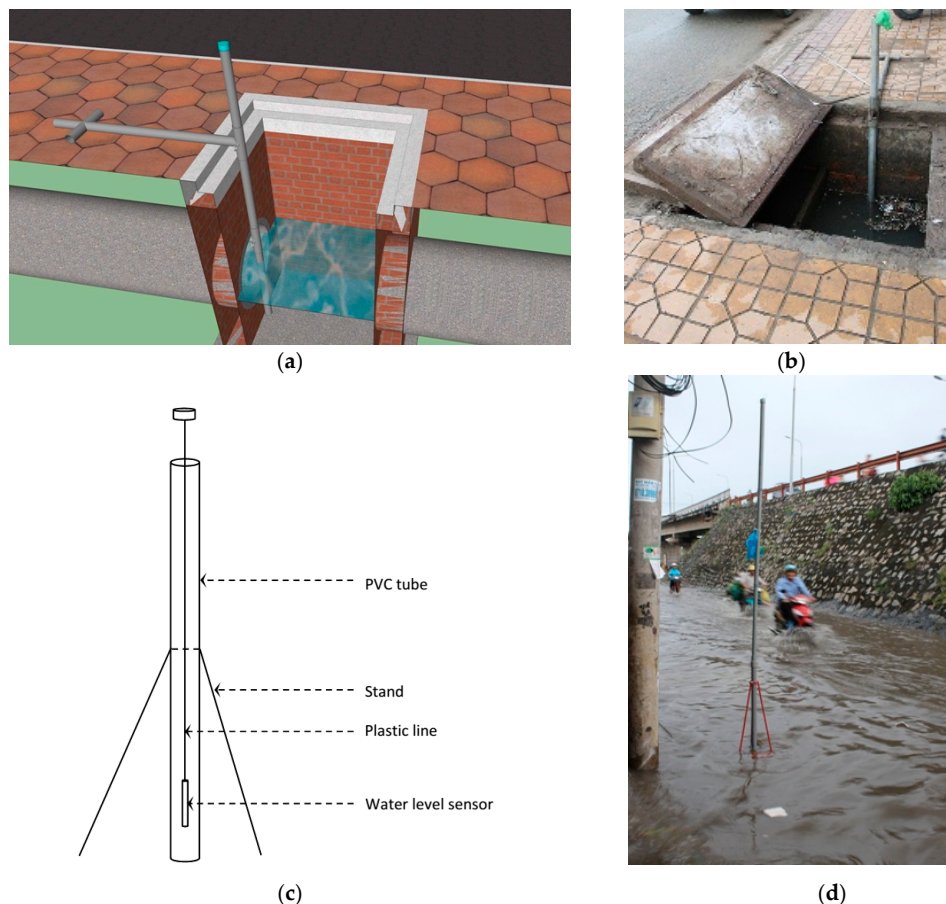
Figure 2. Water level measurement setups to measure the flood depths in sewers (a,b) and in streets (c,d) in Can Tho.
