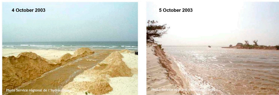
Figure 8. Ground photographs showing the initial trench (4 October 2003), dug on the night of 3 October 2003, across the Languede Barbarie to alleviate flooding of parts of St. Louis. The 5 October 2003 photograph shows the trench considerably widened by river and tidal flow (Photo credit: Service régional de l'Hydraulique, St. Louis du Sénégal).
